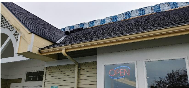
Piles of asphalt shingles await installation on the Community Center roof
